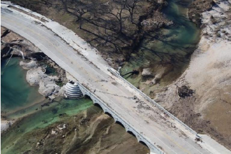
The bridge at Flat Rock Crossing just south of Junction sustained significant damage from the October floods. Because Flat Rock serves as a critical access point in the South Llano River Paddling Trail, the use of the trail is severely limited at this time. The Alliance is working with TPWD to evaluate alternative access points until damage to the bridge can be addressed.
